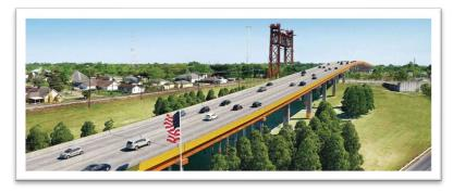
approaches. The main lift span is approximately 150 feet long by 34 feet wide. The main span with the lift towers is approximately 250 feet long.
